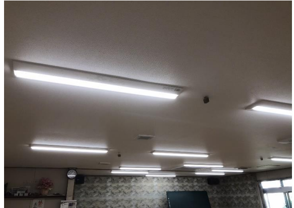
(LED照明工事)
